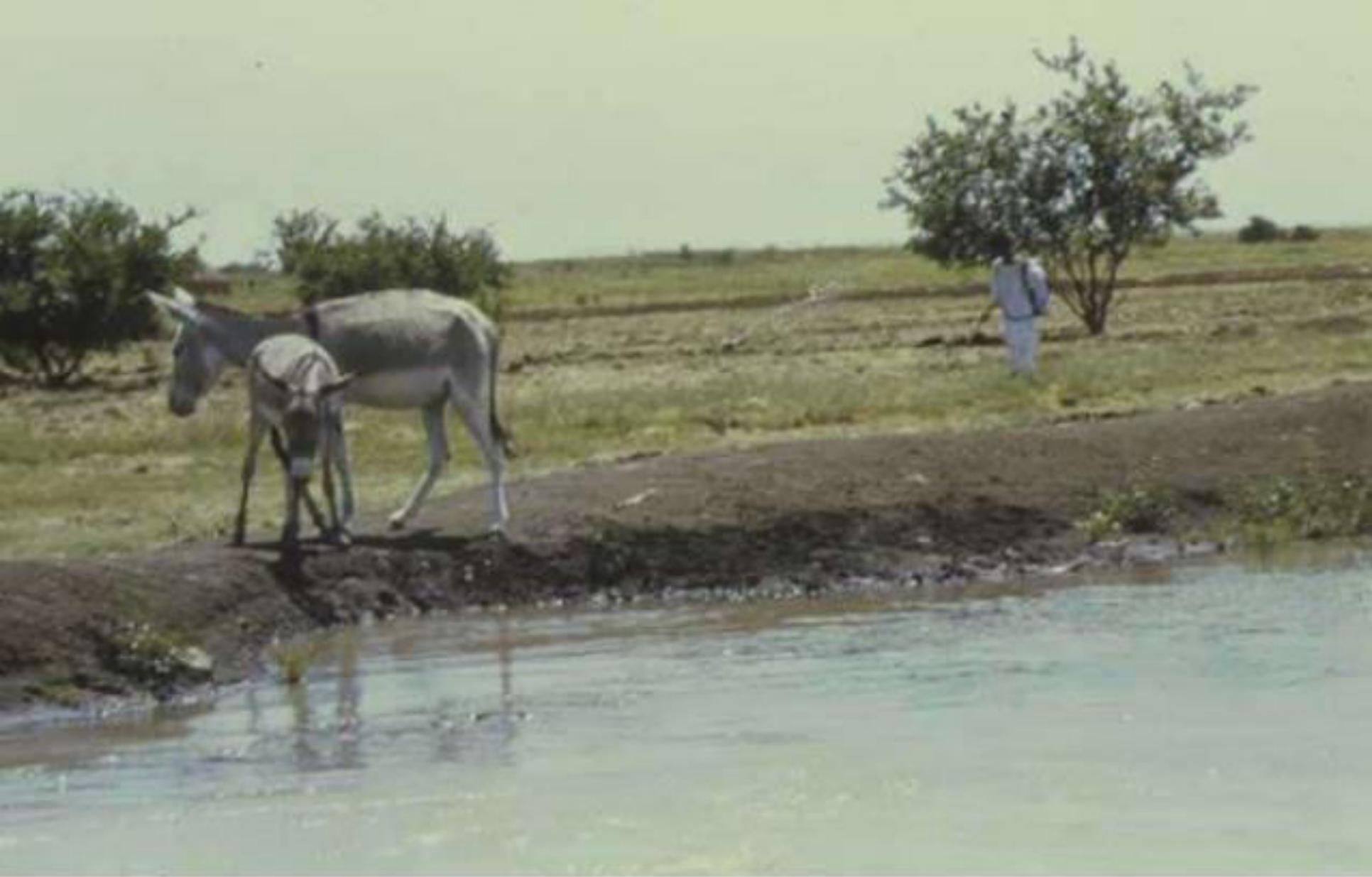
**Canal side breakage due to animal burrowing**
