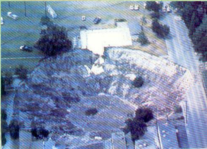
A collapse sinkhole that formed suddenly in Winter Park, Florida, in 1981
