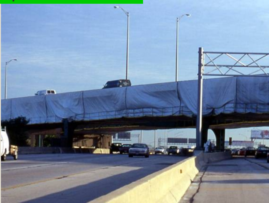
Painting Steel Bridge
