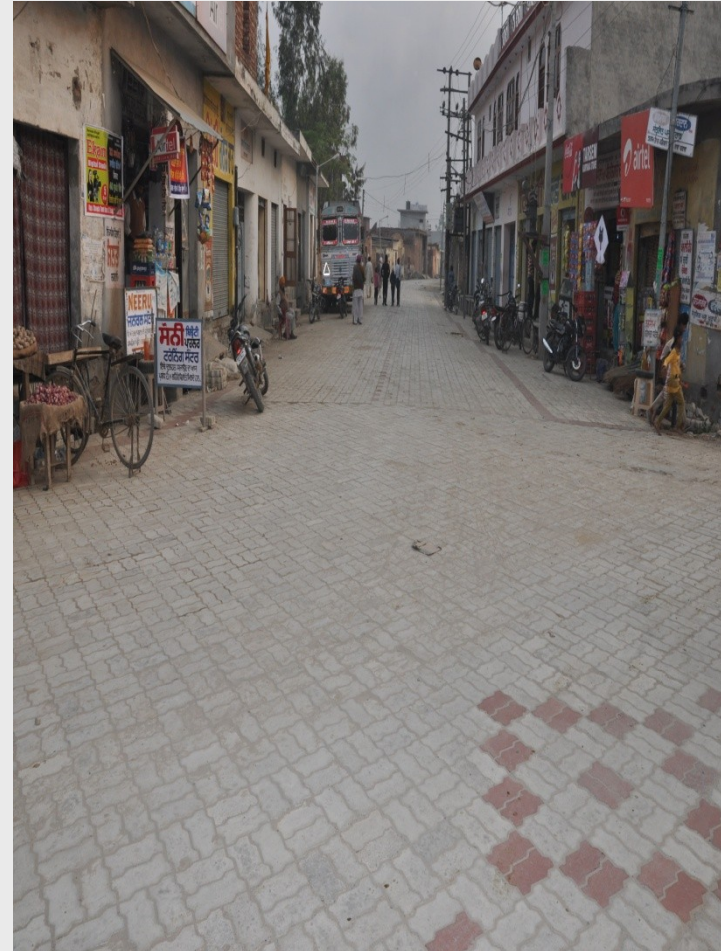
Street after sewer and paver work
