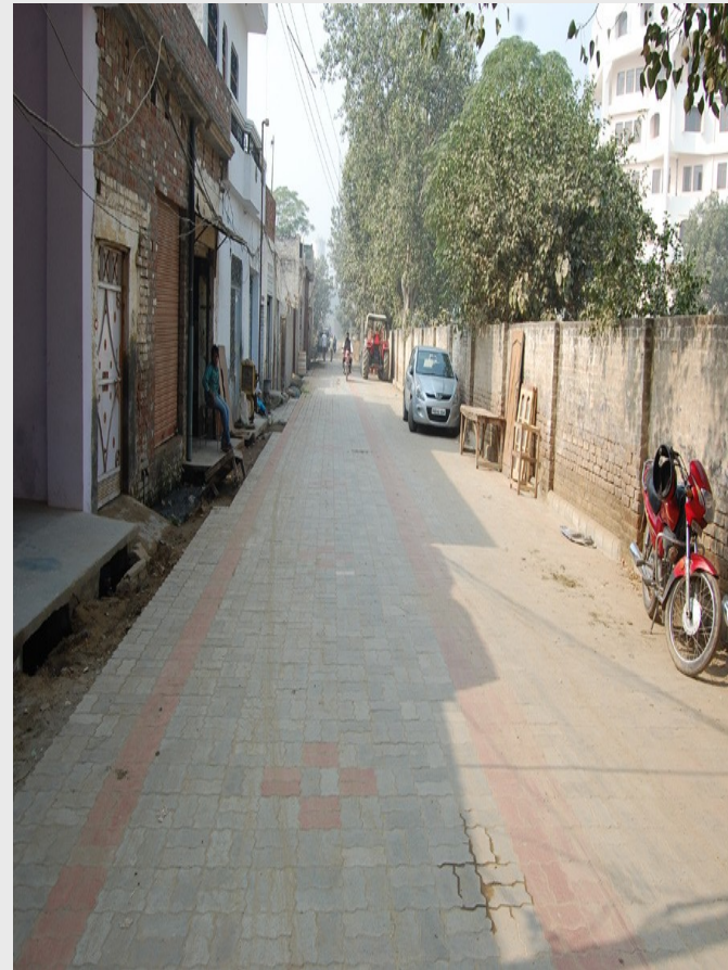
Interlocking Paver after laying of sewer in street
