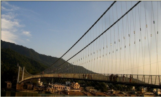
LAXMAN JHULA – RISHIKESH 150 M SPAN (FOOTBRIDGE)
