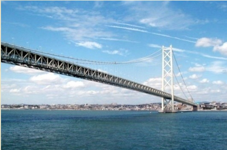
AKASHI KAIKYŌ BRIDGE - JAPAN 1991 M – SPAN
