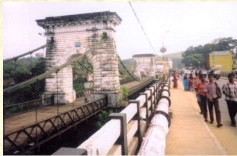
KALLADA RIVER BRIDGE- KERALA
