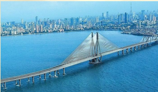
BANDRA WORLI SEA LINK SPAN 40M (5.6 TOTAL LENGTH)
