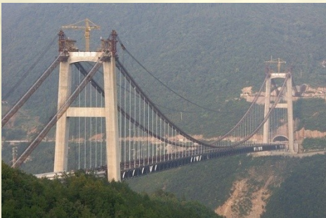
SIDU RIVER BRIDGE – CHINA (1222 M SPAN)
