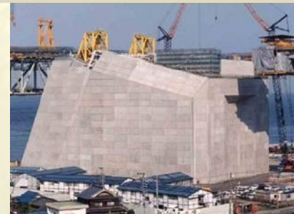
Fig. 31 Anchorage 4A of Akashi-Kaikyo bridge.
