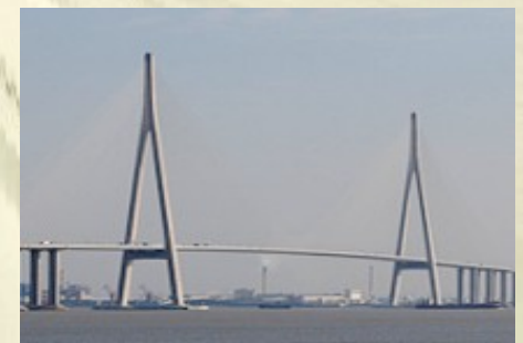
SUTONG BRIDGE - CHINA 1088 M SPAN
